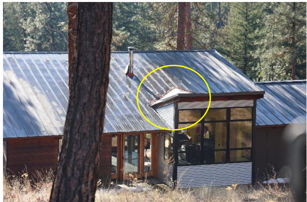
This unique design has allowed for needle cast to accumulate.
